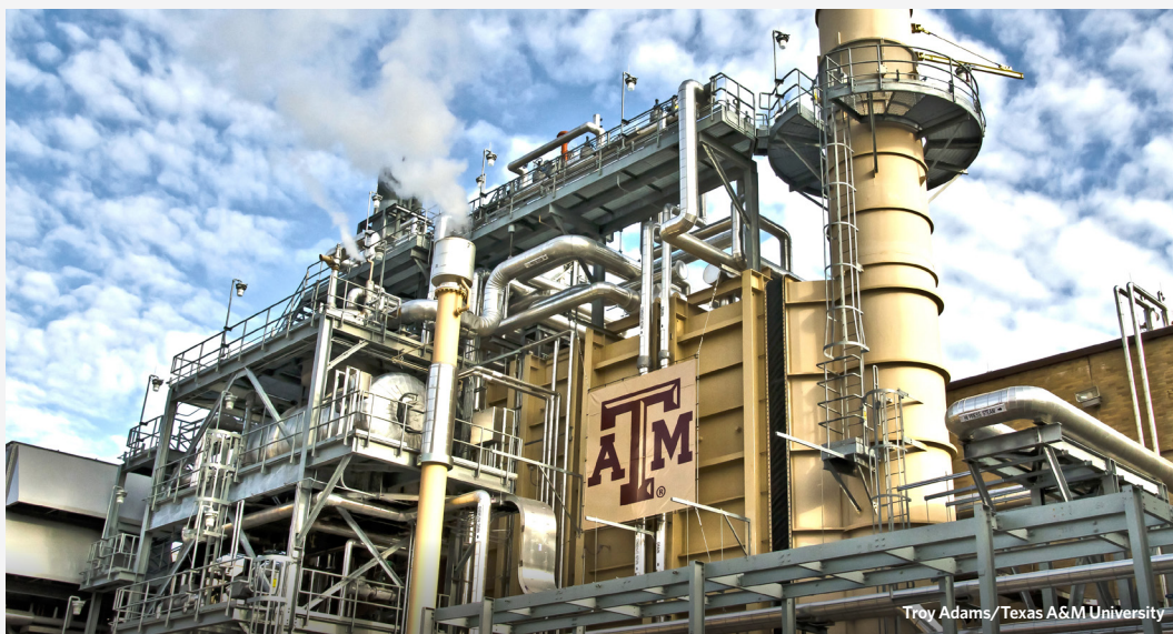
Combined heat and power system at Texas A&M University.
