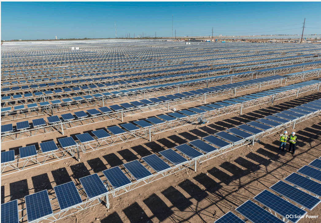
The Alamo 4 Solar Farm in Bracketville.
