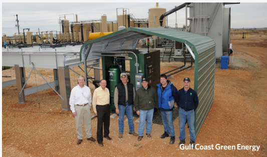
Waste heat to power installation at a South Texas natural gas field.
