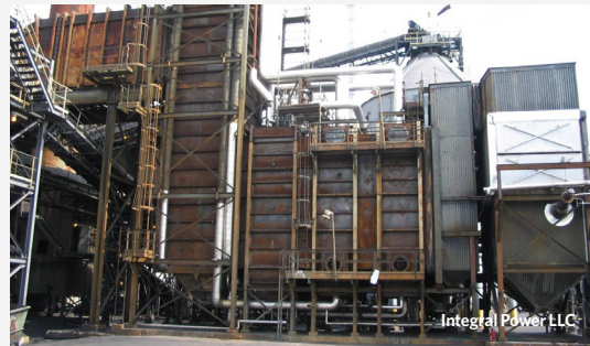
Industrial energy efficiency project by Integral Power.
