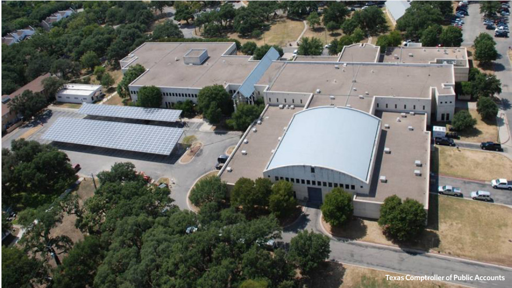
Solar photovoltaic system on a carport at Camp Mabry.
