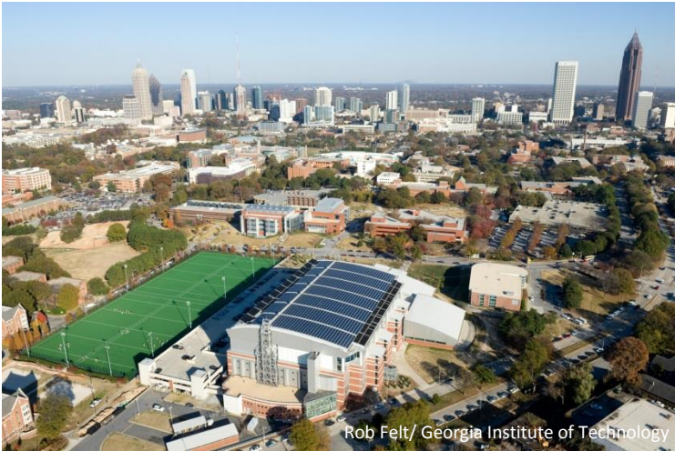
Rooftop solar at Georgia Tech's campus recreation center
