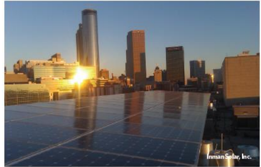
Photovoltaic project built by Inman Solar.
