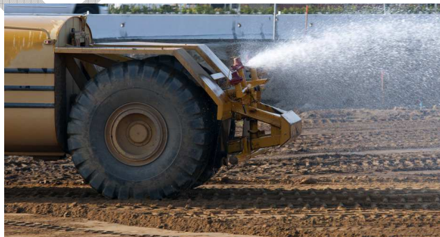
Figure 15: Spraying water can reduce construction dust
