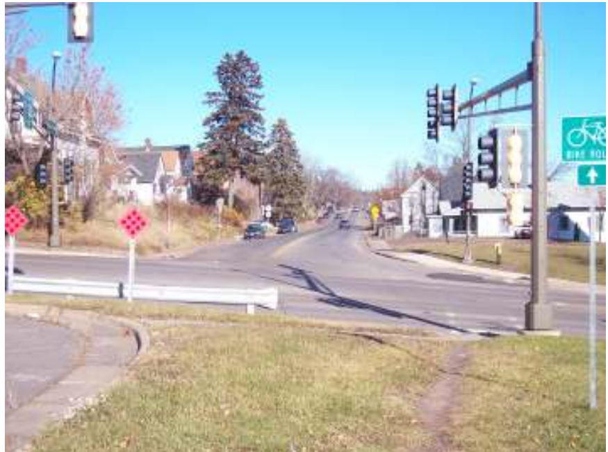
Looking east across Sixth Avenue East at Ninth Street
