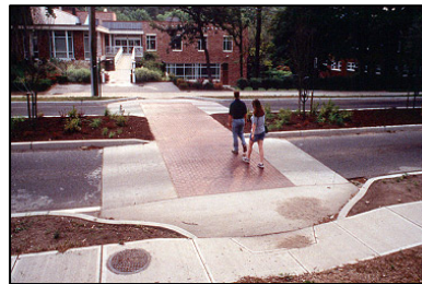
Elongated Speed Humps and Raised Crosswalks
