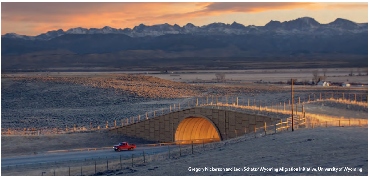
Each year, thousands of mule deer and pronghorn safely move across U.S. Highway 191 near Pinedale, Wyoming, via this overpass and adjacent underpasses.
