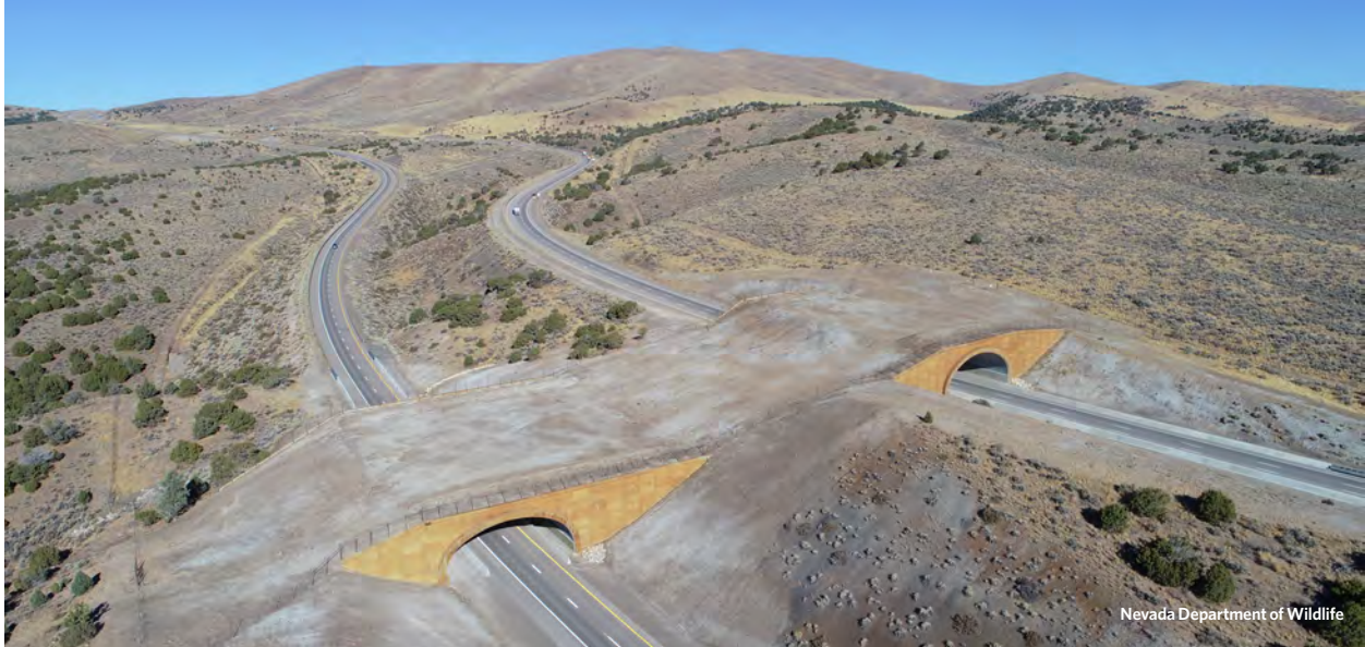
Overpasses, such as this one built along Interstate 80 in Nevada for mule deer, provide safe passage for wildlife.
