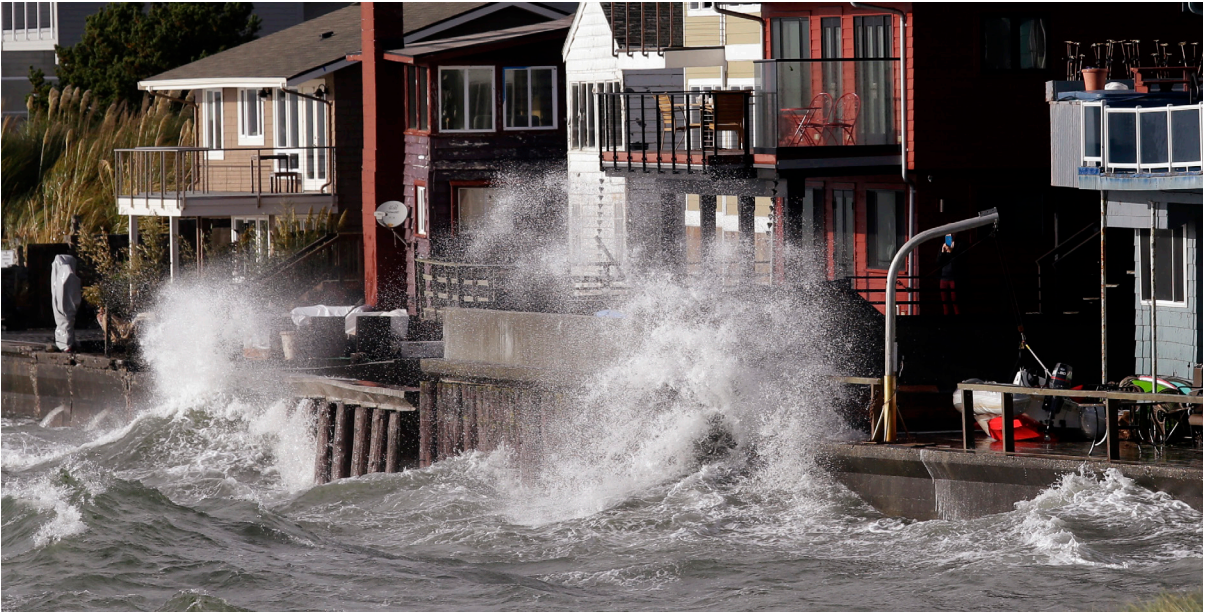
Waves batter a sea wall in Seattle after a heavy storm in October 2016. Although sea walls can protect properties, they can also multiply the force of waves onto surrounding areas, creating problems elsewhere and leading to calls to reduce their numbers. Elaine Thompson/AP Photo
